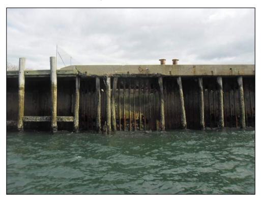
Figure 20: View of perforated steel bulkhead along Dry Dock #4.
