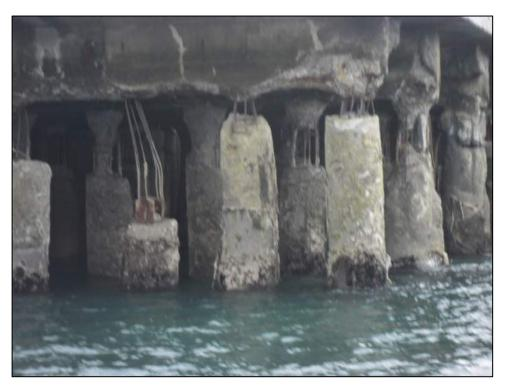
Figure 14: Typical condition of piles supporting the North Jetty wharf deck.
