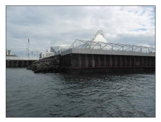
Figure 21: Overall view of recent steel bulkhead and riprap repairs at Wharf 8.
