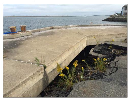
Figure 16: View of open sinkhole in the deck of Dry Dock #4.
